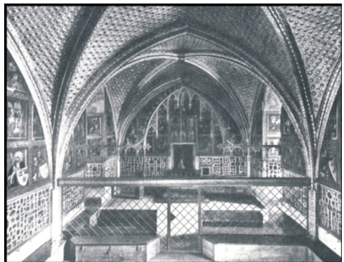
Fig 14: Chapel of the Holy Cross. View into the presbytery on the north side of the second story of the large tower.
