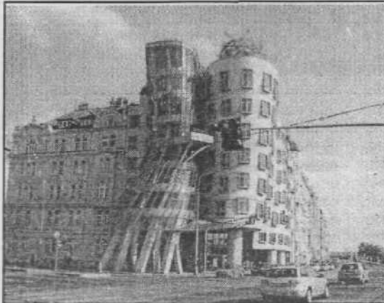
Figure 8: The Dancing House on Rašín embankment
