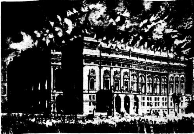
Fig. 4 Destruction by fire, 1881
